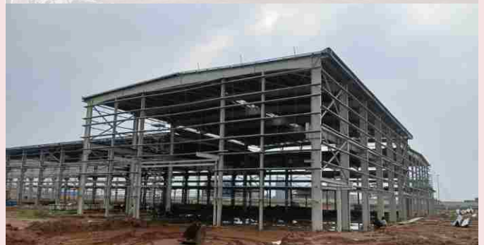
Ratnamani metal & tubes ltd (Factory Building)
